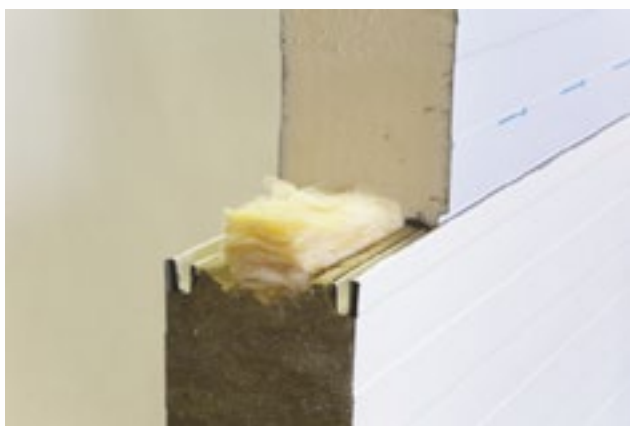
Photo. No. 2. View of the connection (overview)
