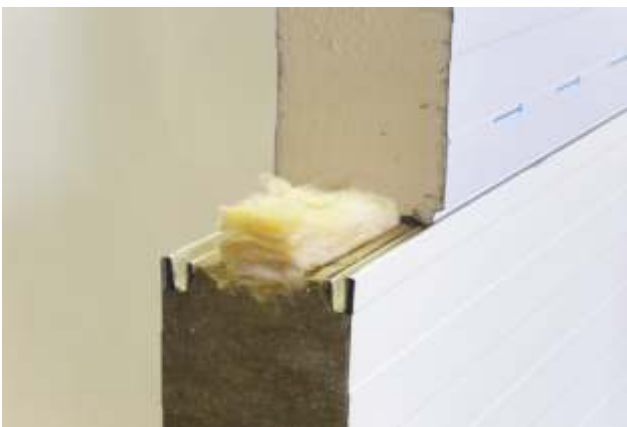
Photo. No. 2. View of the connection (overview)
