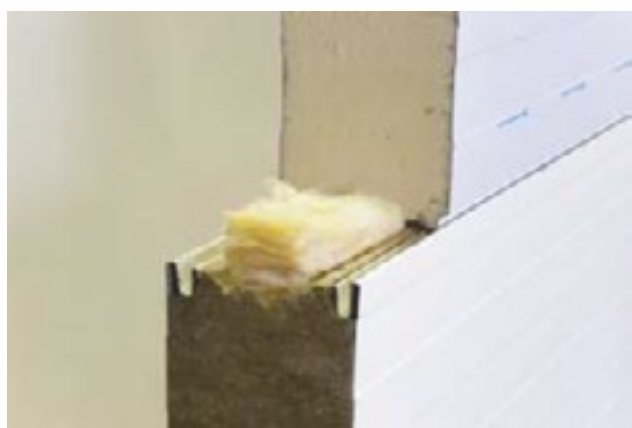
Photo. No. 2. View of the connection (overview)
