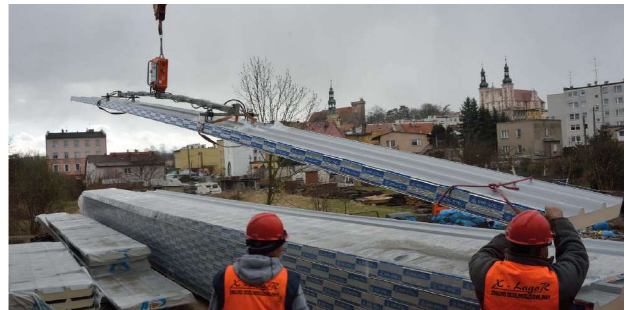
Photo 6. Lifting a roof panel from a stack.
