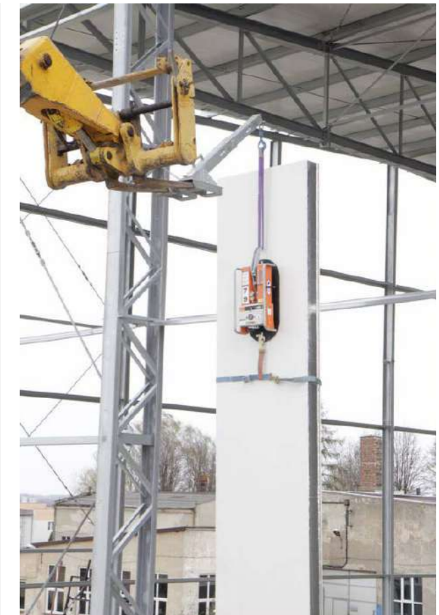
Photo 11. Vertical installation of sandwich wall panels.
