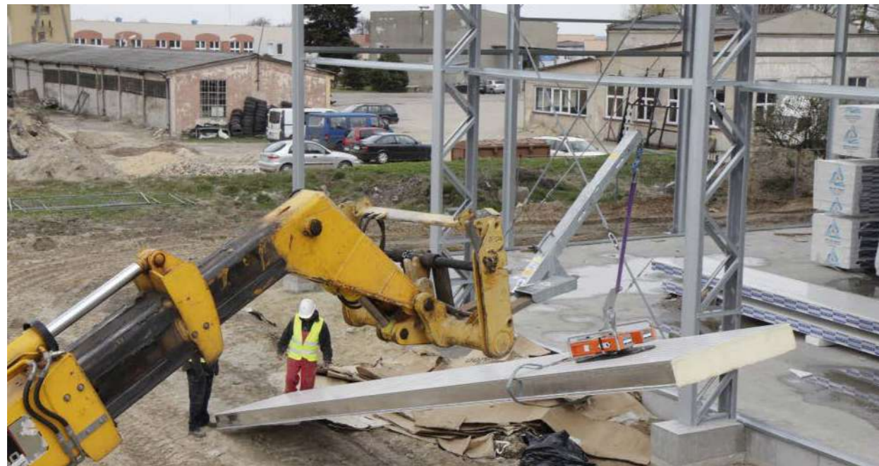
Photo 10. Lifting a panel with a vacuum suction cup (vertical installation).
