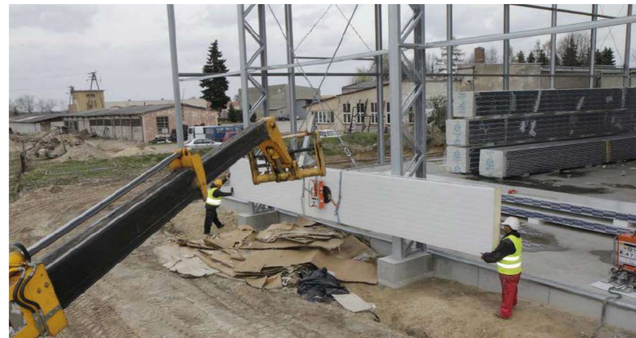
Photo No. 9. Horizontal installation of wall sandwich panels.
