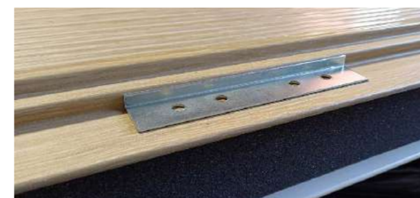
Photo no. 12. Position of the PM1 washer in the lock of the panel with a concealed fastener.
