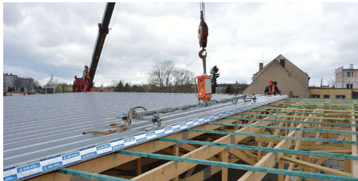
Photo 7. Laying roof panels on the building structure
