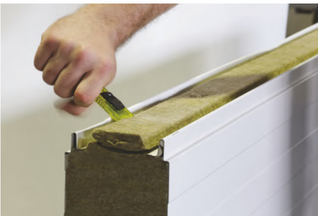
Photo. No. 3. Suggested way to remove the GS MW plate tongue
