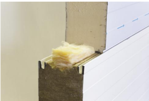
Photo. No. 2. View of the connection (overview)
