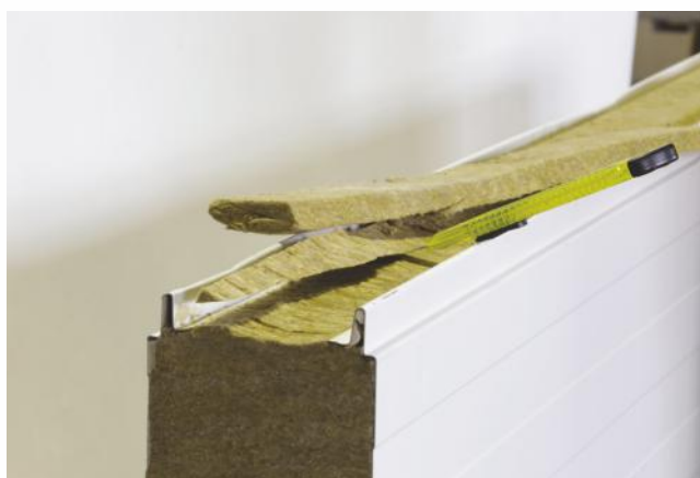
Photo. No. 3.P Suggested way to remove the GS MW plate tongue
