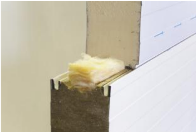
Photo. No. 2. View of the connection (overview)
