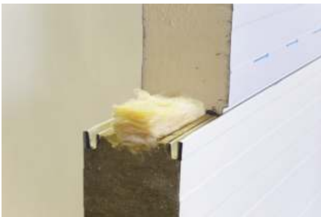
Photo. No. 2. View of the connection (overview)
